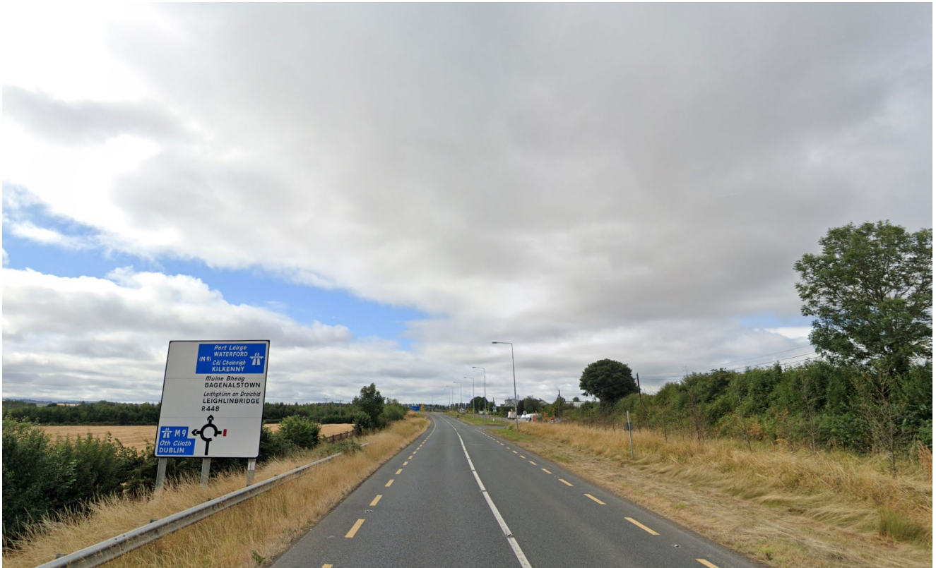
Plate 6-1: Link 1 – R448 Kilkenny Road (Facing South): Source Google Street View Aug '18 (52.773425, -6.953526)
