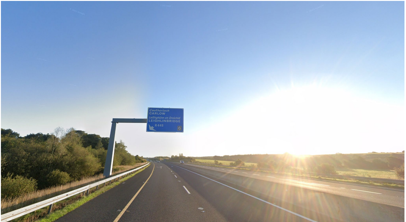
Plate 6-6: Link 2a – M9 Jn.6 Northbound Off-slip (Facing North): Source Google Street View Sept '22 (52.766473, -6.961483)
