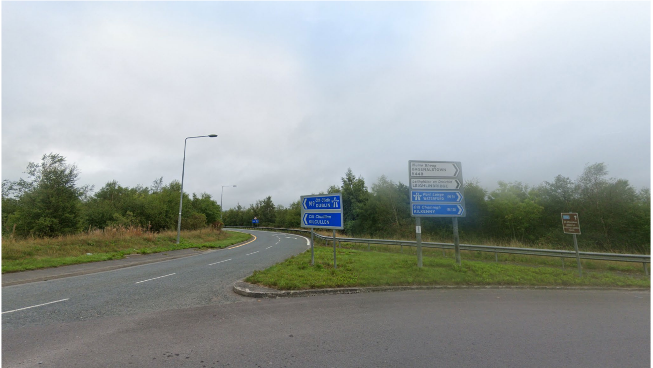
Plate 6-8: Link 2b – M9 Jn.6 Northbound On-slip (Facing North): Source Google Street View Sept '22 (52.770857, -6.953514)
