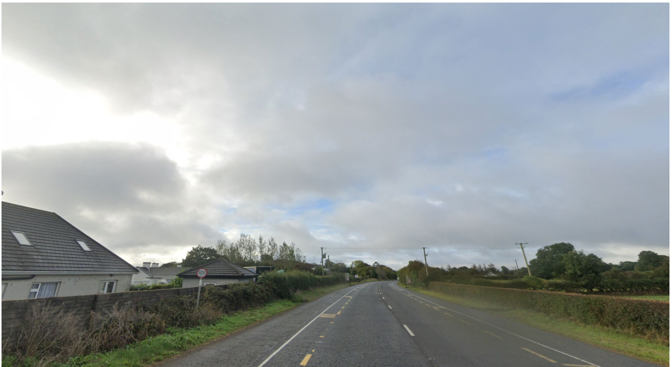
Plate 6-4: Link 11 – R448 Nr. Royal Oak Rd. (Facing South): Source Google Street View Sept '19 (52.708879, -6.982321)
