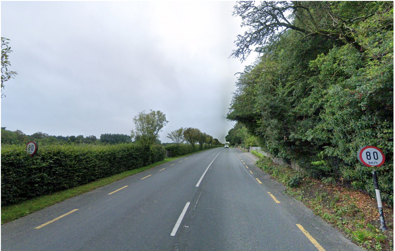
Plate 6-12: Link 15 – R705 Leighlinbridge (Facing North): Source Google Street View Sept '22 (52.738314, -6.975090)
