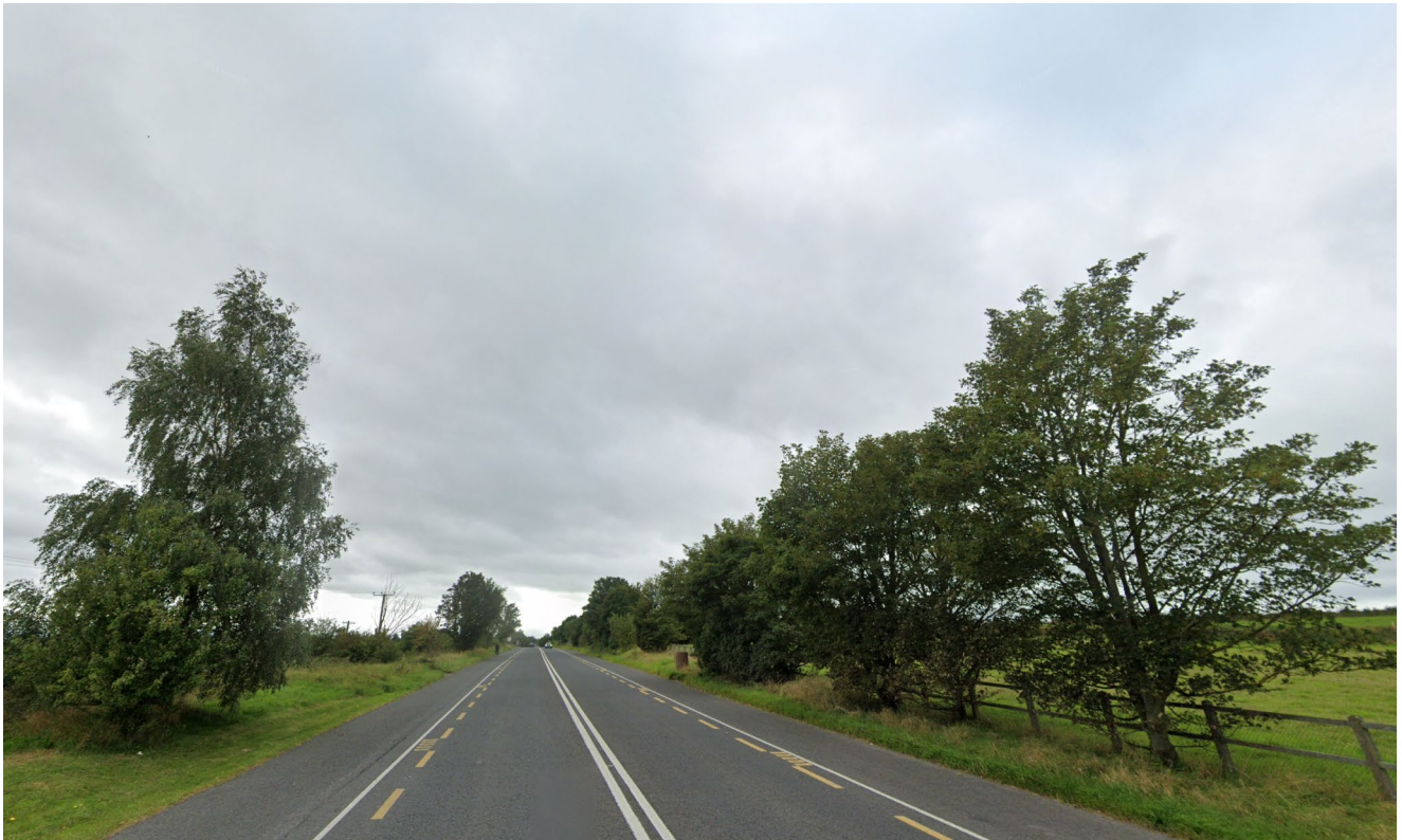
Plate 6-5: Link 12 – R448 South of R724 (Facing South): Source Google Street View Sept '19 (52.699702, -6.987978)
